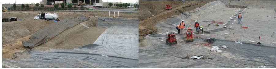
Inspection of clay under geomembrane
